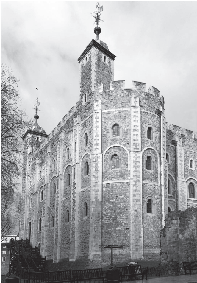
Figure 12.4. View of the apse from the south-east (Photo: Roland Harris).
