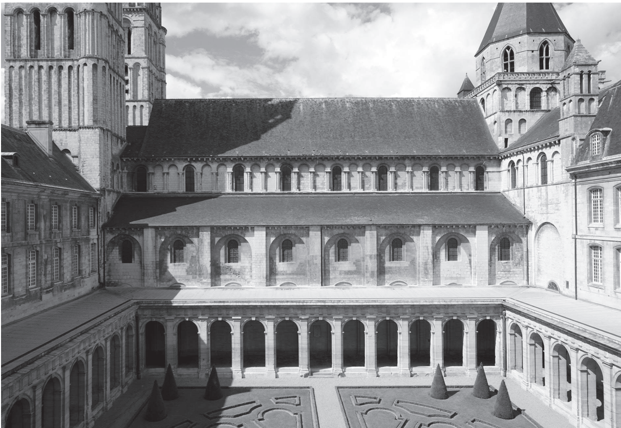
Figure 12.12. St Etienne, Caen, south side of nave showing arcading surrounding the gallery-level windows (Photo: Roland Harris).
